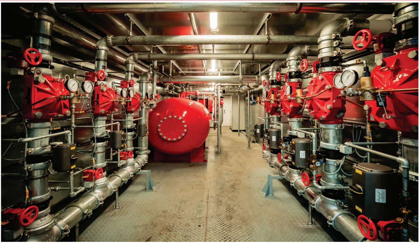
Fire Water Valve Houses
